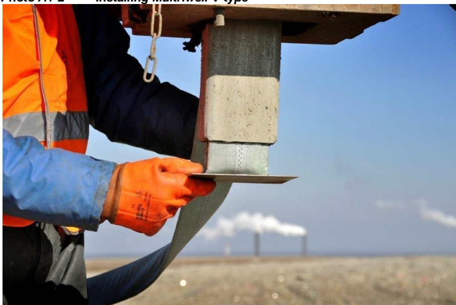
Photo A1-2 Installing Multriwell V-type
