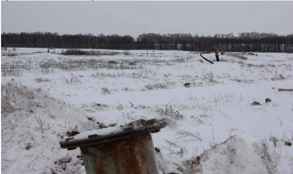
Figure A6-2 Old non-functioning vertical LFG extraction wells
