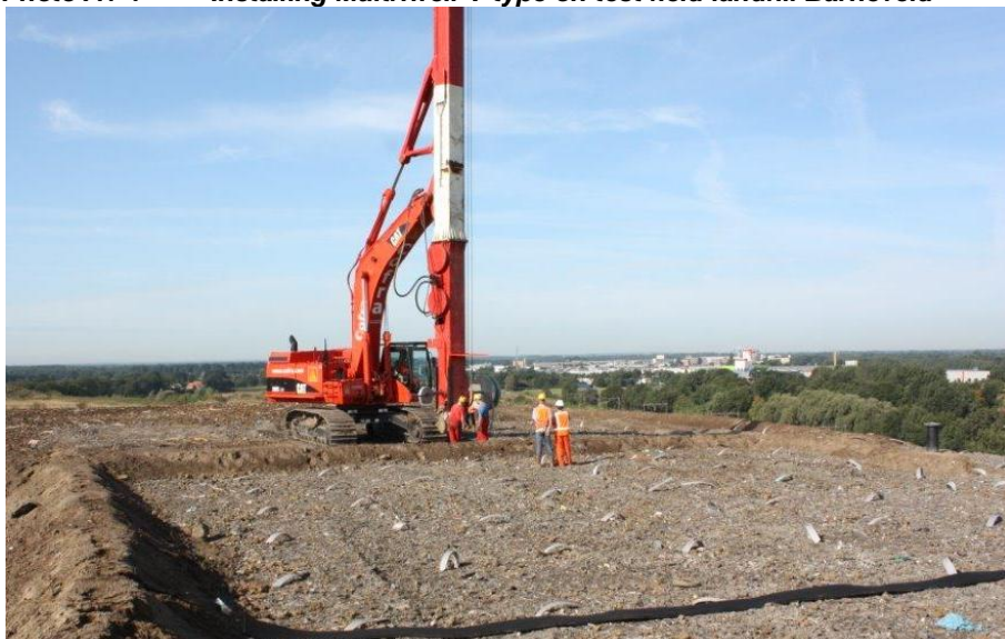
Photo A1-1 Installing Multriwell V-type on test field landfill Barneveld
