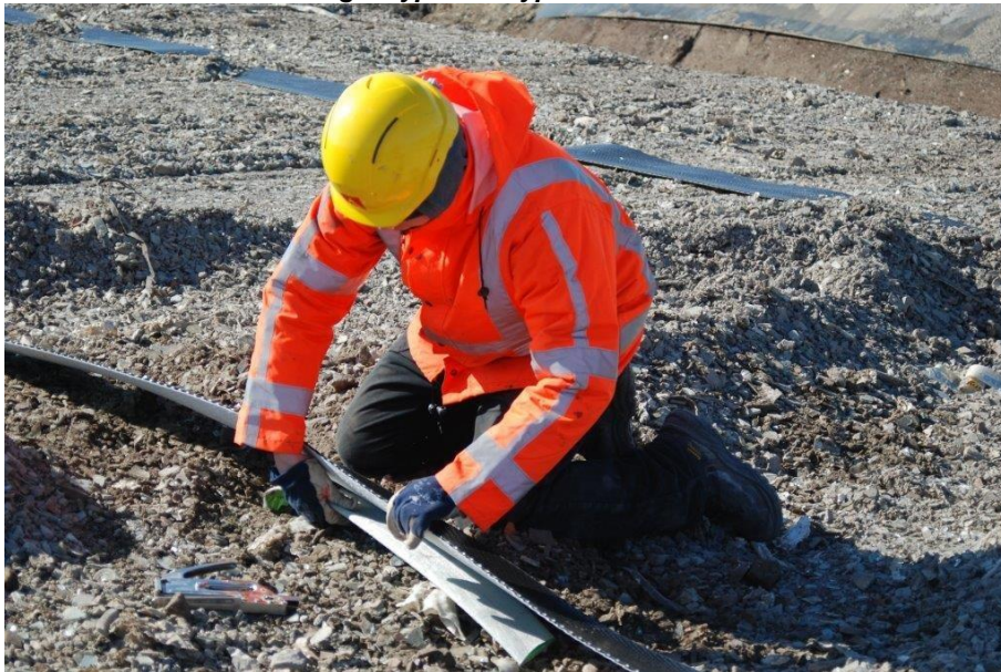
Photo A1-4 Connecting H-type to V-type
