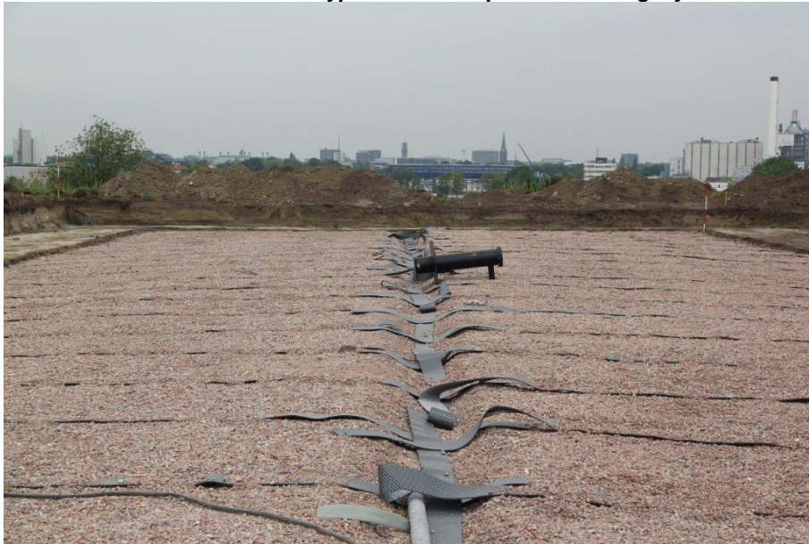
Photo A1-6 Overview of H-type and Put on porous levelling layer
