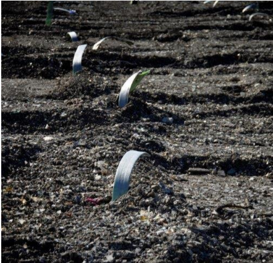
Photo A1-3 Installed Multriwell V-type
