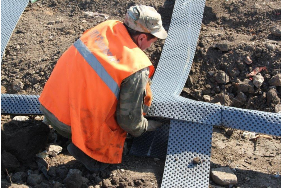
Photo A1-5 Connecting H-type to perforated collector drain
